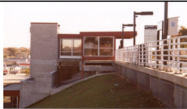
Former Pennsylvania-Reading Seashore Line Absecon station. The station was built in 1962.
