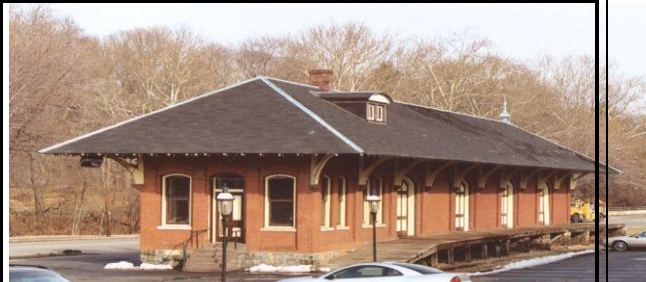
CNJ freight station at Bethlehem, PA.
