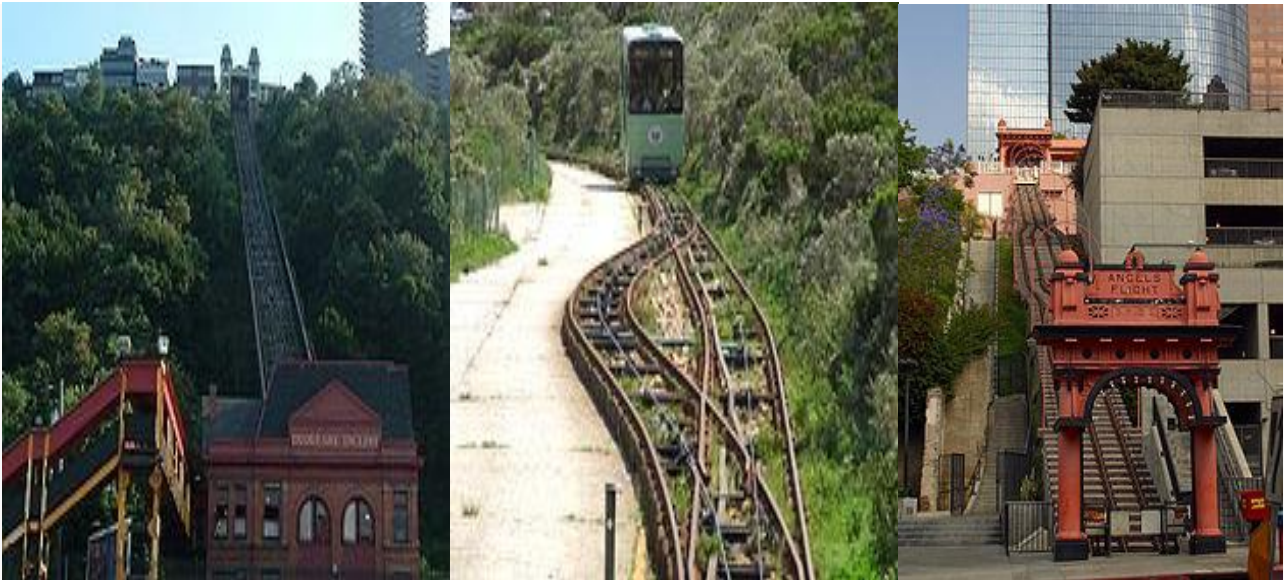
Duquesne Incline, Pittsburgh, Pennsylvania, U.S., with full-length parallel tracks Passing track with Abt switch on the Flying Dutchman Funicular at Cape Point, South Africa Angels Flight, Los Angeles, USA, three-rail configuration with passing track
