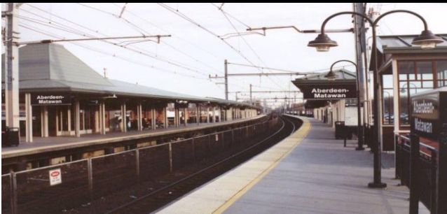
The new Matawan station is built along a curve as seen in 2011.
