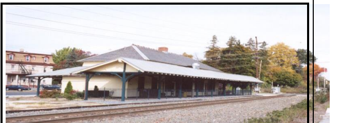
Woodbury station. The station has been restored and is now a restaurant.
